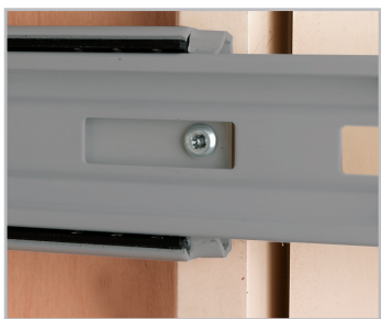
Front of slides mount to the face frame of the cabinet
